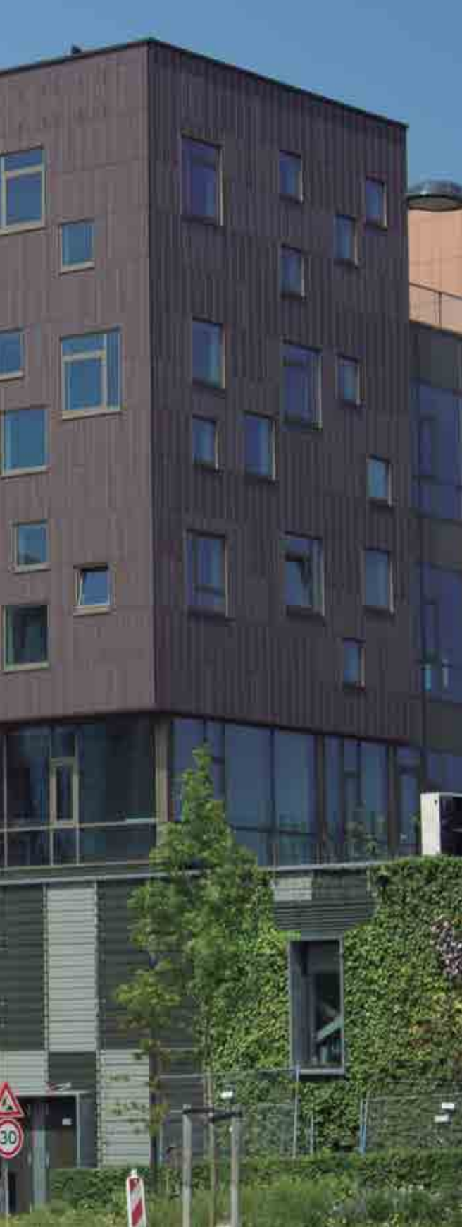
Proyecto/ Project : Taurusavenue Building. Amsterdam (Netherlands)
